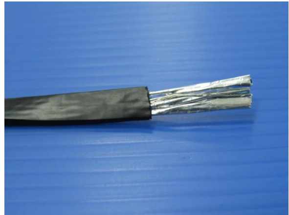
2. Strip and removed 20mm of jacket.
